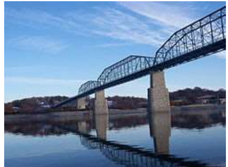
Chattanooga Pedestrian Bridge
