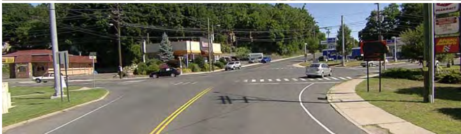
View on Route 63 from South of the Intersection
